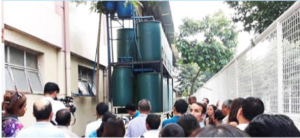
Marikina City. Public schools like H. Bautista Elementary School use rainwater harvesting systems (RHWs) to collect water for watering plants, cleaning rooms and flushing toilets. RHWs alleviate the impacts of climate change on water security.
