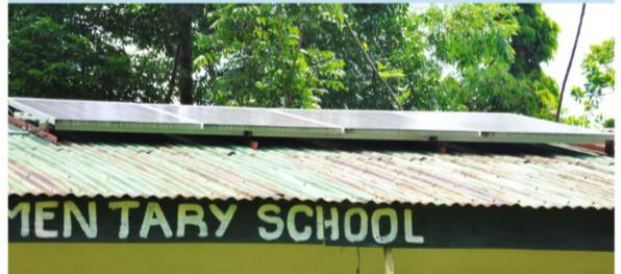
Kalayaan, Laguna. The GreensPH and Green Earth Resolution installed a two-kilowatt solar panel and electrical system in the remote island community of Pulot-Bay, which now energizes the Pulot-Bay Elementary School.
