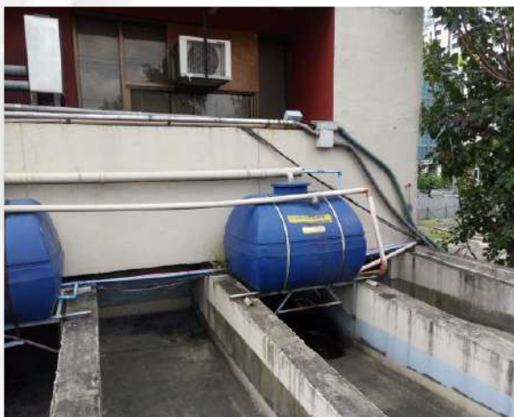
Mapúa Makati's rainwater collector tanks
