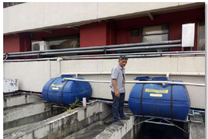
Mapúa Makati's rainwater collector tanks
